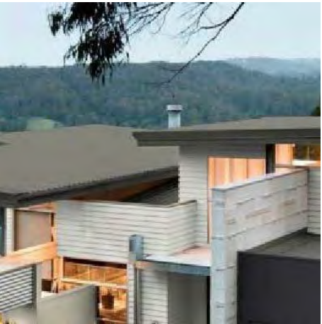
4. ROOF SHEETING - WALLABY COLORBOND
